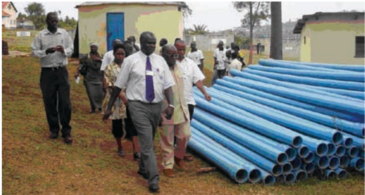
Area Manager Masaka Inspects mains extension pipes with visitors from Tanzania
