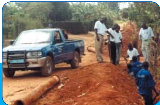
Typical pipe laying exercise, Kampala
