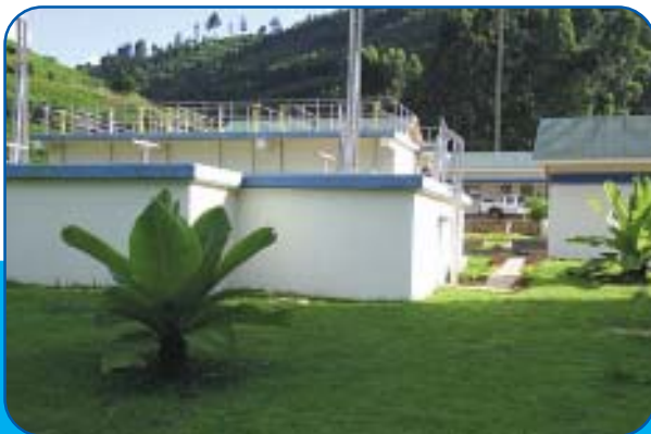
Kiyora Water Works, Kabale
