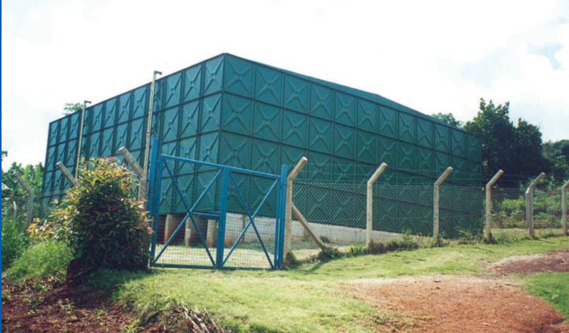
A post stressed steel storage reservoir on Mutungo Hill in Kampala
