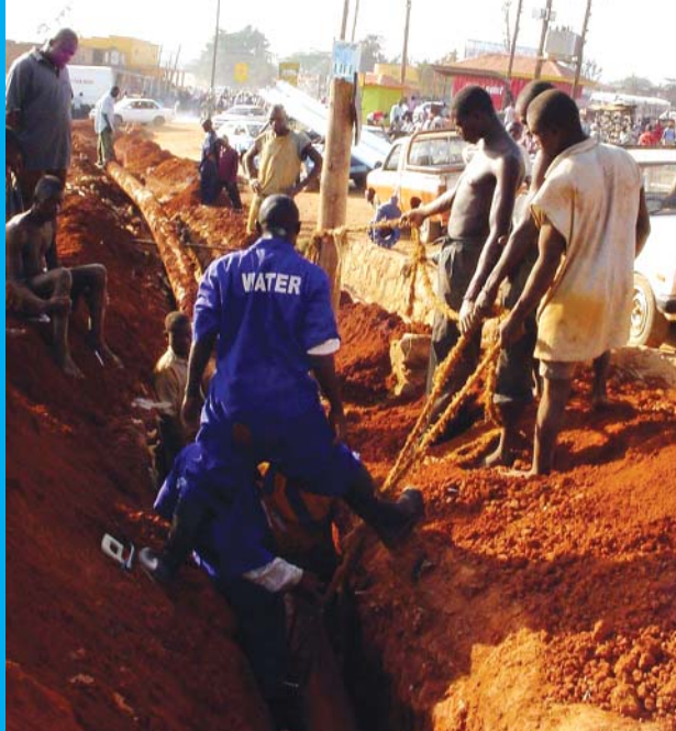
Katigondo mains extension work in progress in Masaka
