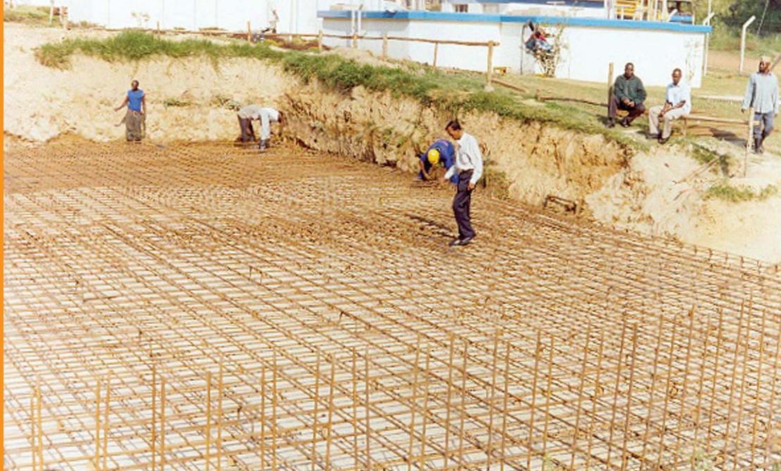
Construction of a reservoir at Kiyooro, Kabale
