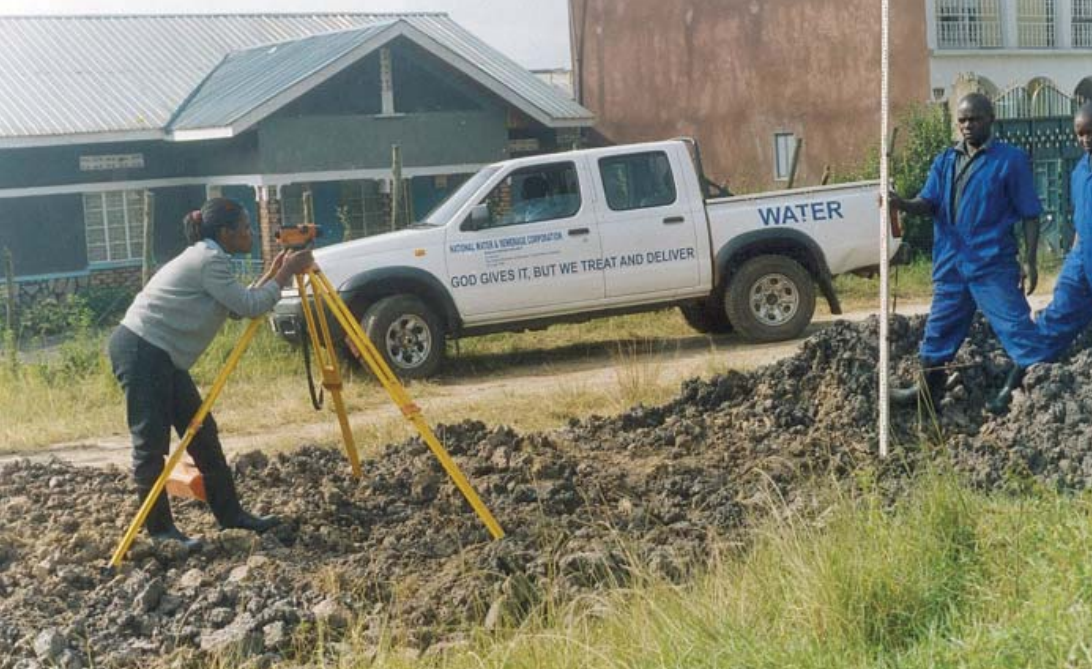
Pipe laying in Kabale
