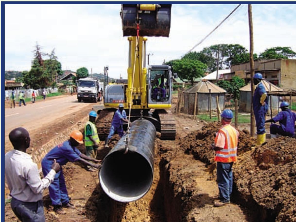
Laying of the new Transmission Mains in progress along Gaba Road
