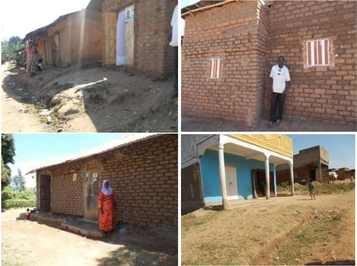
Photo 4: Some structures likely to be affected by the proposed project
