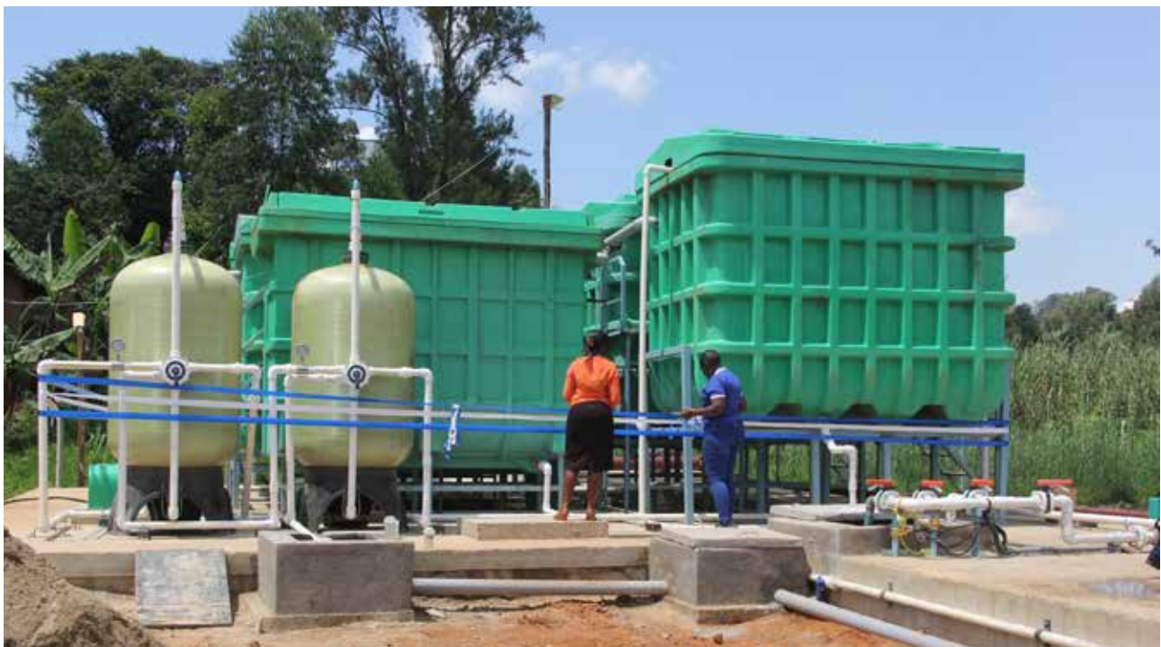
Compact sewerage treatment units installed and functional
