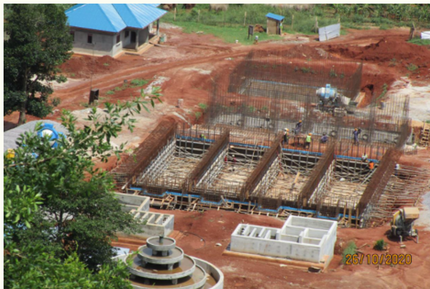
Ongoing reinforcement and concrete works on the Project for upgrading of Kapeeka Water Supply System
