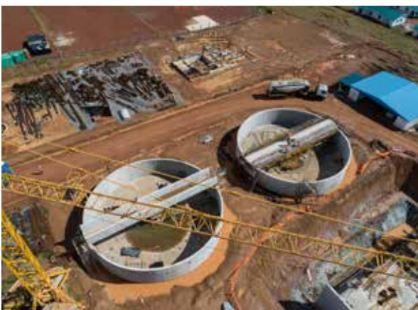
Water filters under construction at Katosi
