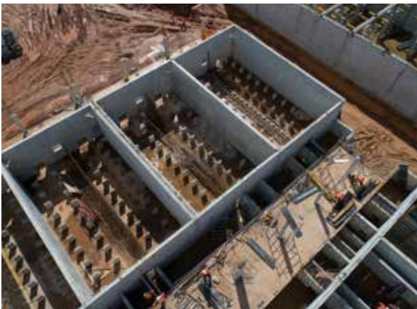
Water filters under construction at Katosi
