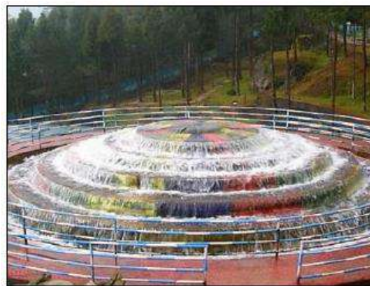
Figure 3-5: An example of a Cascade Aerator
