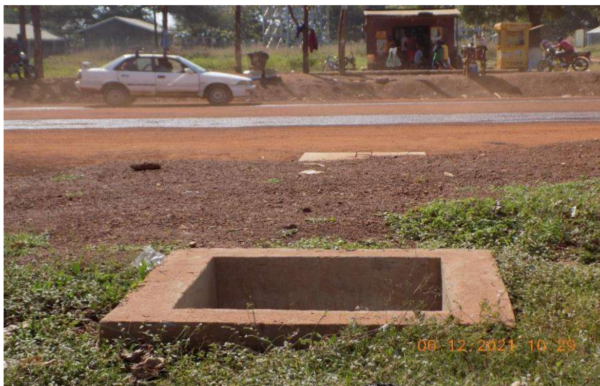
Figure 9-10: Structures for pipe crossings provided by the Contractor on Atiak – Adjumani – Laropi
