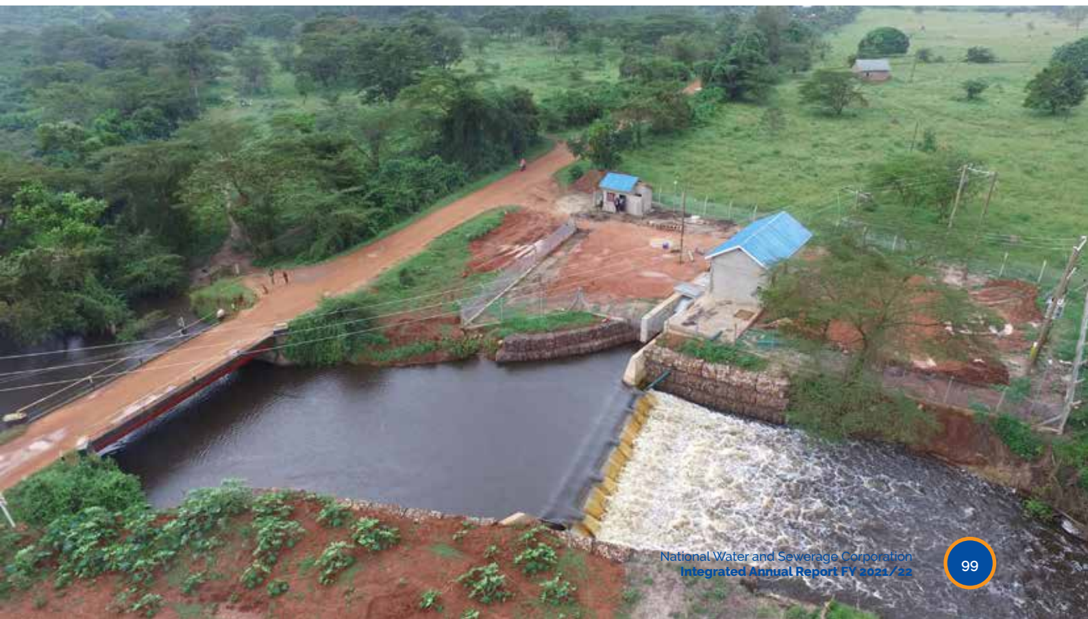
Kapeeka Water Treatment Plant.
