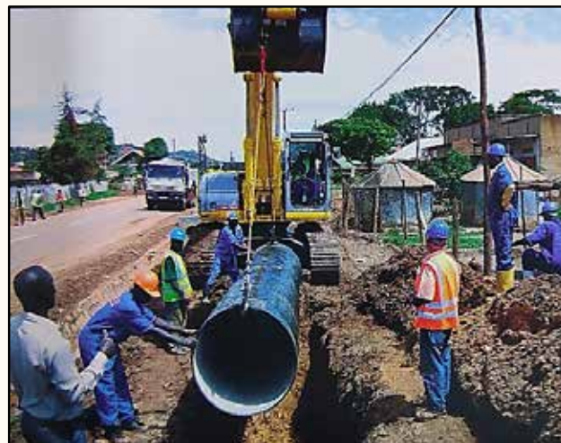
New Transmission Main from Gaba Treatment Plant
