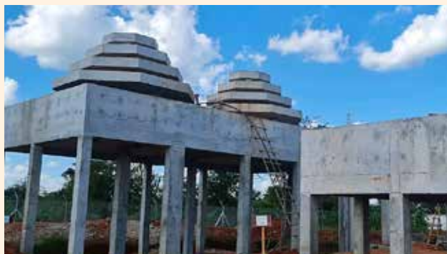
Aerators at the new Lyantonde Kakyere Water Treatment Plant
