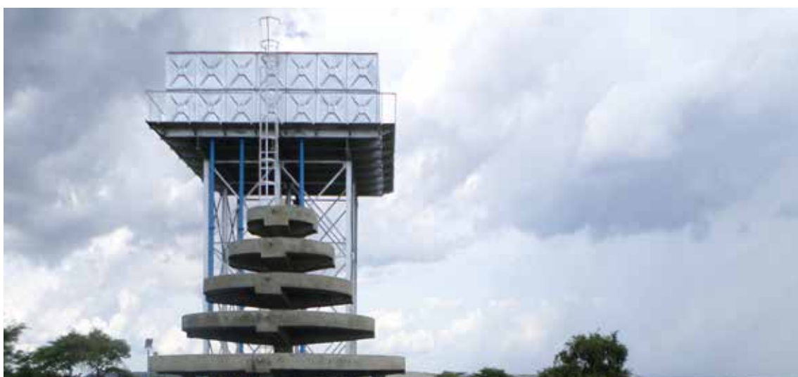
Aerators at the Lyantonde Kakyere Water Treatment Plant.
