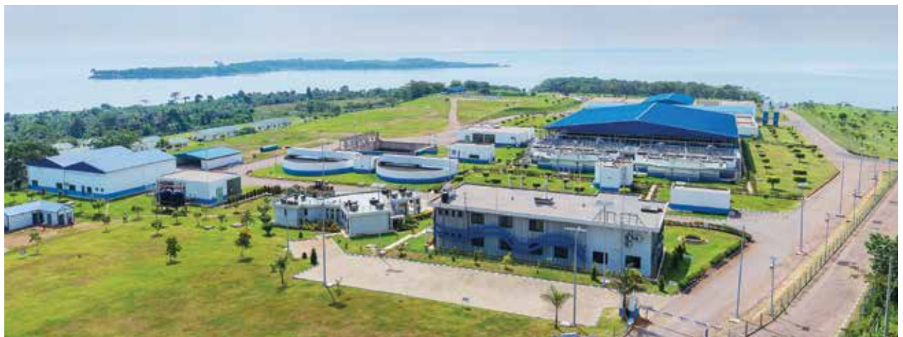
Katosi Water Treatment Plant
