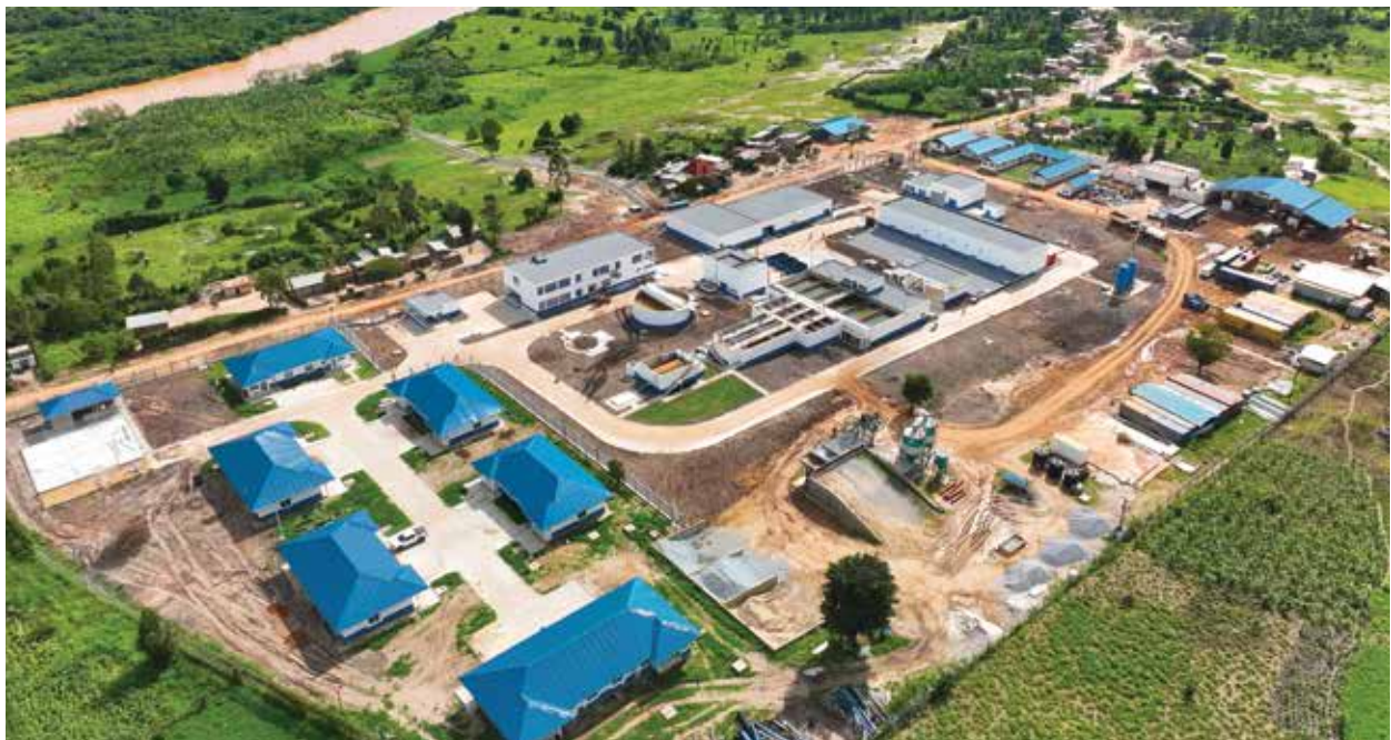
Kagera Water Treatment Plant under the South Western Cluster Project
