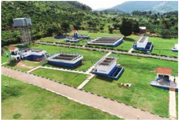
Kapeeka Water Treatment Plant - Augumented Project
