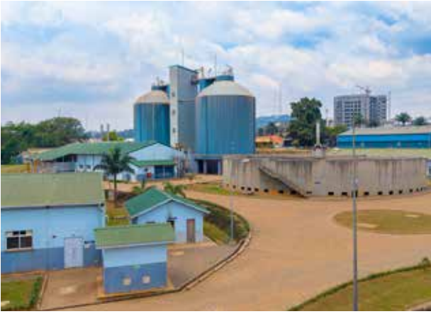
Nakivubo Wastewater Treatment Plant
