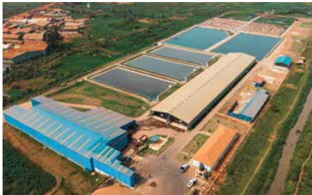
Nalukolongo Wastewater Treatment Plant
