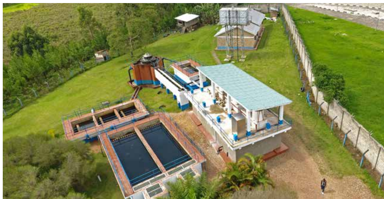
Nyaruzinga Water Treatment Plant - Bushenyi
