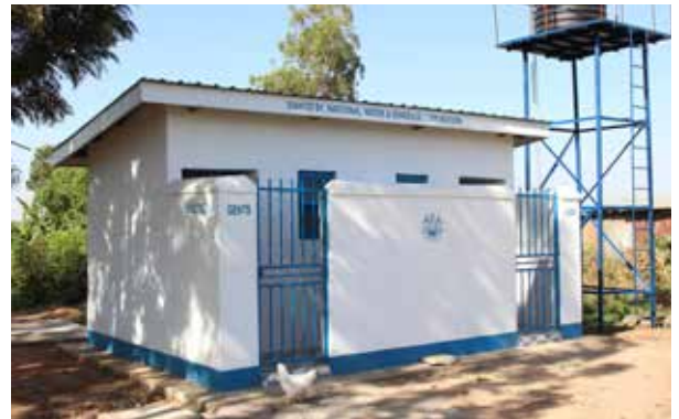
One of the Toilets Constructed in Tororo Area under CSR
