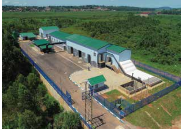
Kinawataka Wastewater Pre-Treatment Plant
