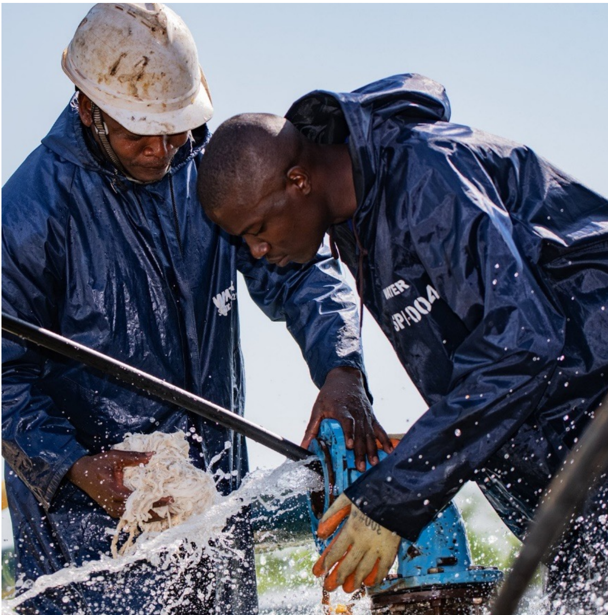
NWSC Staff working on a pump to ensure continuous service delivery.
