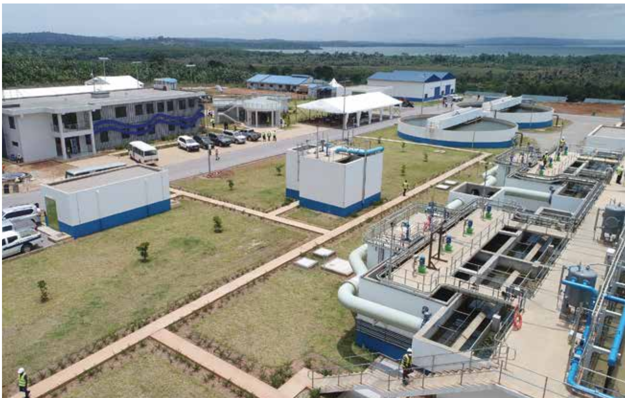
Katosi Water Treatment Plant
