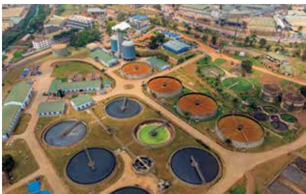
Nakivubo Wastewater Treatment Plant
