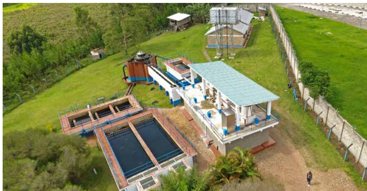
Nyaruzinga Water Treatment Plant - Bushenyi
